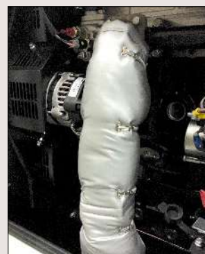
FASCIA COIBENTE INSULATION JACKET
